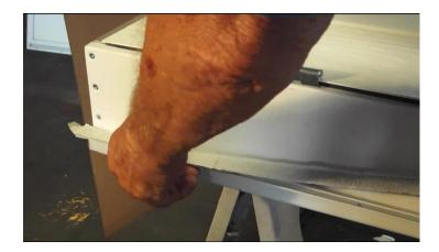
1. Making certain all mounting surfaces (siding seams included) are securely fastened and flat around the perimeter of the rough opening. There should be no obstruction in the opening (i.e. nails, staples, nailing strips, belt rails, etc.). 2. Apply sealant tape to the backside of the door's mounting flange, covering all screw holes.
