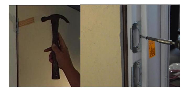
8. If the gap between the jamb and stud is greater that ¼" and if the jamb is bowed out at the lock, it will be necessary to shim behind the jamb.
