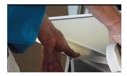
1. Making certain all mounting surfaces (siding seams included) are securely fastened and flat around the perimeter of the rough opening. There should be no obstruction in the opening (i.e. nails, staples, nailing strips, belt rails, etc.). 2. Apply sealant tape to the backside of the door's mounting flange, covering all screw holes.
