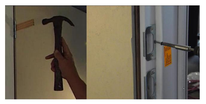
8. If the gap between the jamb and stud is greater that ¼" and if the jamb is bowed out at the lock, it will be necessary to shim behind the jamb.
