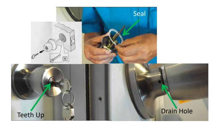
7. When installing the door lock, place the seal on the exterior of the door, and position the door lock where the teeth of the key are pointing up when inserted into the lock. The drain hole will be at the bottom when installed properly.
