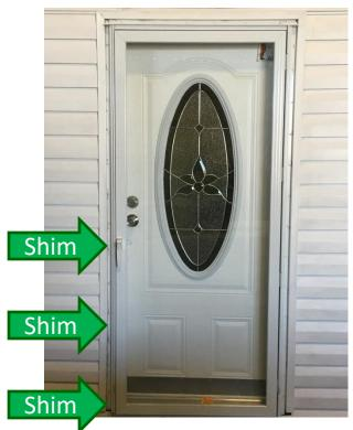
3. <u>Do NOT open the door or remove shipping clips</u> <u>or shims before installation.</u> Opening the door before installation will destroy the proper squaring of the door. If shims are not in place for the storm door, position one shim in the striker location and another 2/3 the way down. Position a third shim on the inside core under the sweep and butting against the lock side jamb.
