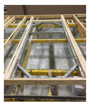
Use OSB or other sheathing on both sides and above door. This will provide stability and structural integrity for the door.
